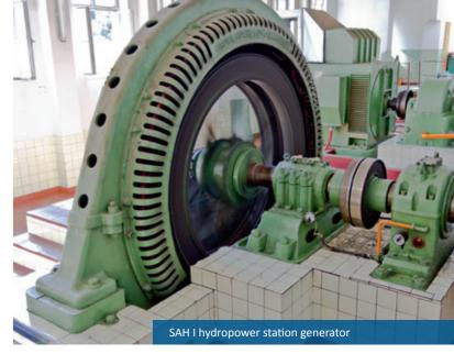
In-house production at the plant's own hydropower station is  $CO_2$ -free. The SAH I hydropower station has a nominal power of 1,500 kW. The associated plant sewer system was extensively rehabilitated from March to August 2020. The rehabilitation increased the efficiency of hydropower generation by up to 5 percent.
